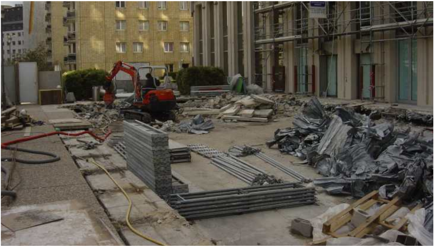
demolition double dalle
